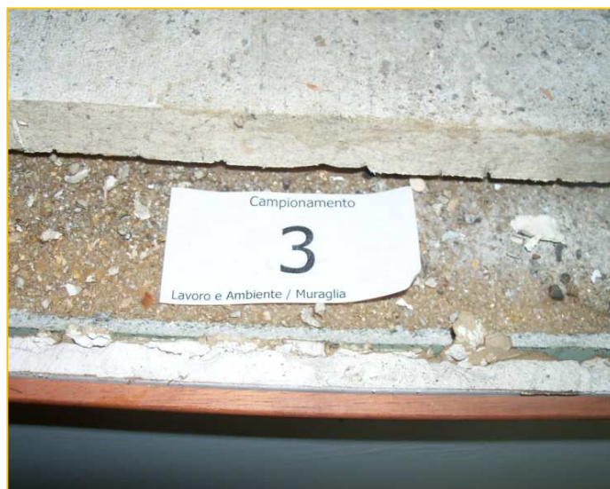
Pannello sandwich in cemento-amianto
